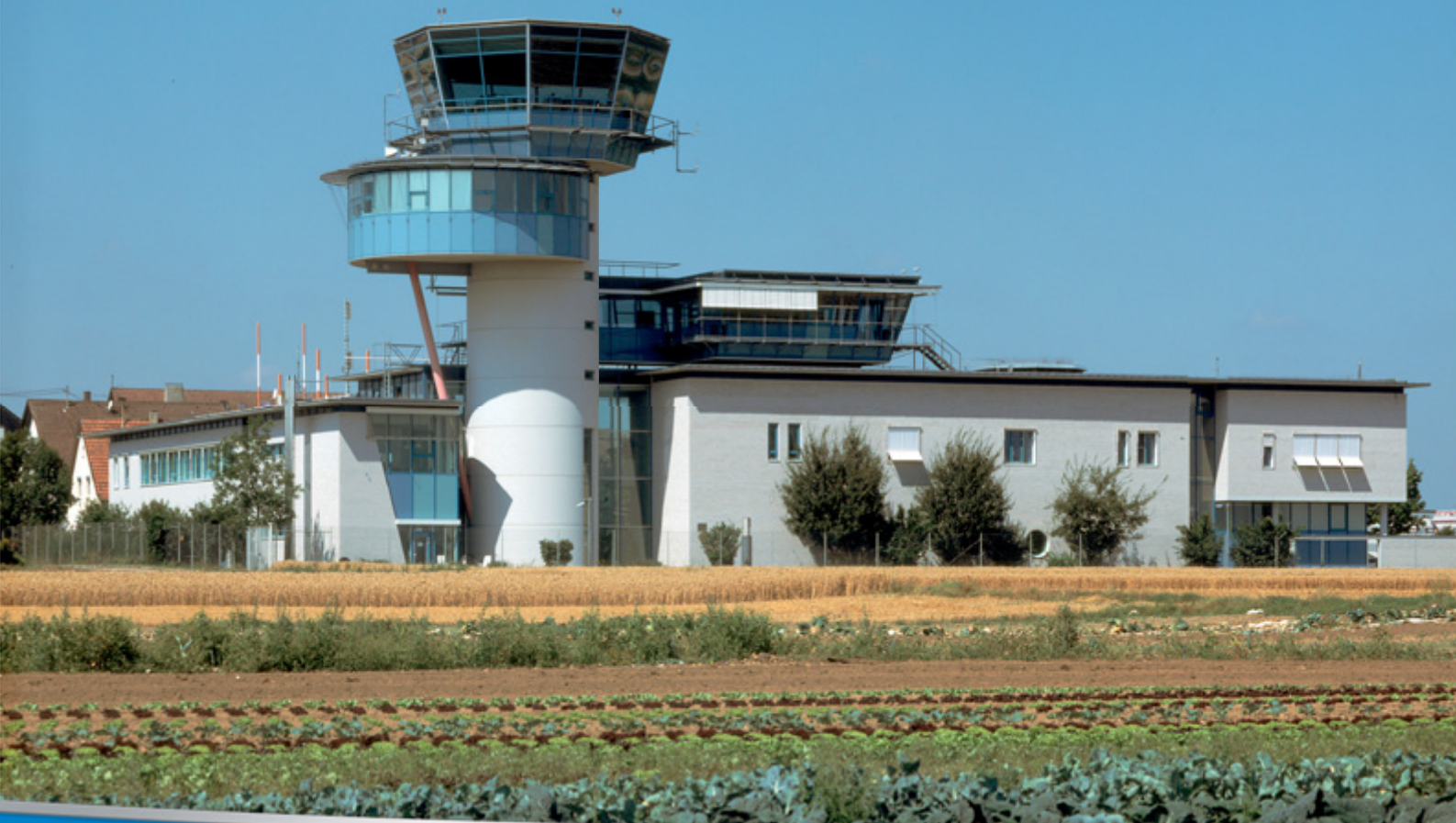
→ Tower Stuttgart. Photo: DFS
